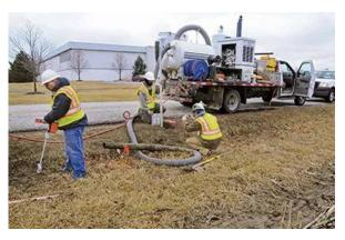
For example, a problem locate resulting from a missing or broken tracer wire can be remediated by installing a new tracer wire. A problem locate resulting from an inaccurate map/documentation can be resolved by properly locating, marking, verifying, and updating the map. This service utilized over time can fundamentally improve a client's utility asset mapping and improve the ROI on programs like One Call Locating and Damage Prevention Vehicles.
